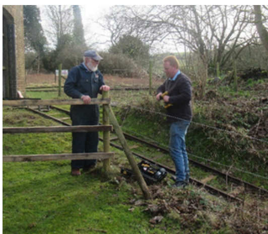
Chris and Matthew working on the new fencing for the incline.
