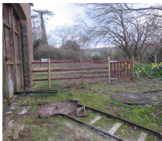
The finished result showing the new access gate.
