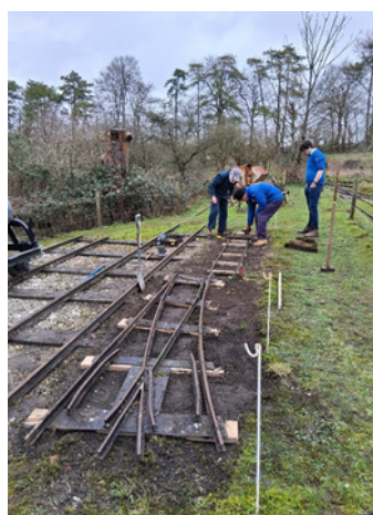
Replacing sleepers in the wagon display area.
